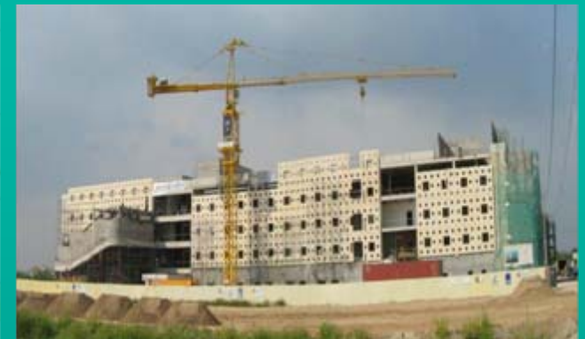
RMIT Vietnam Saigon South Construction
